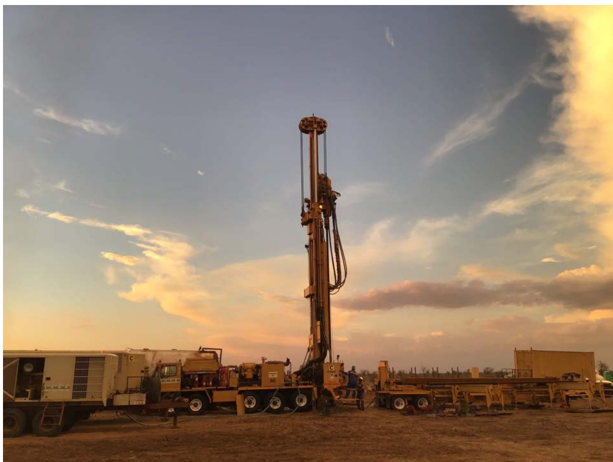
Drilling Operations at Tlou Energy's Lesedi CBM Project, Botswana – November 2018
