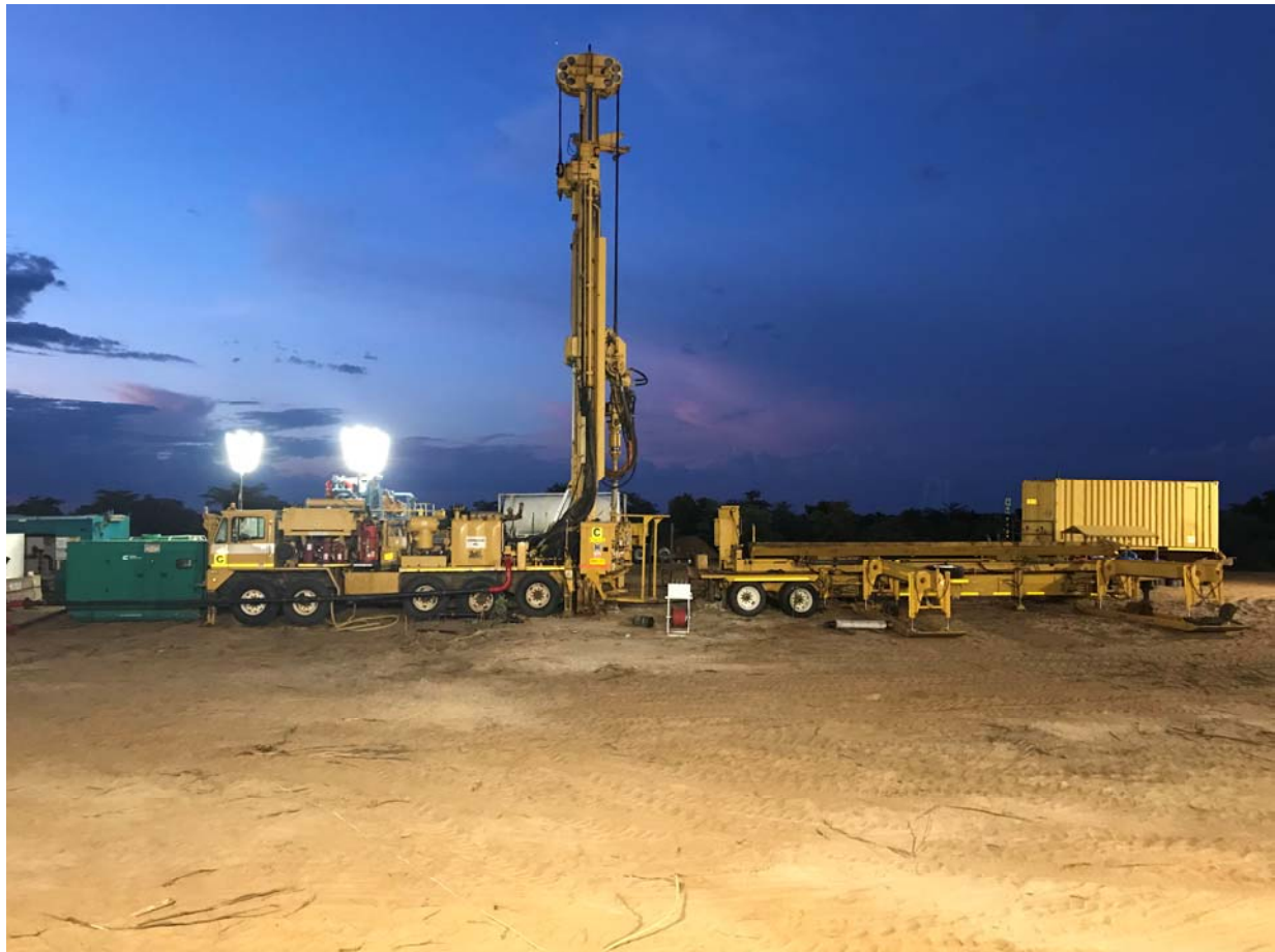
Lateral well drilling, Lesedi CBM Project – January 2019
