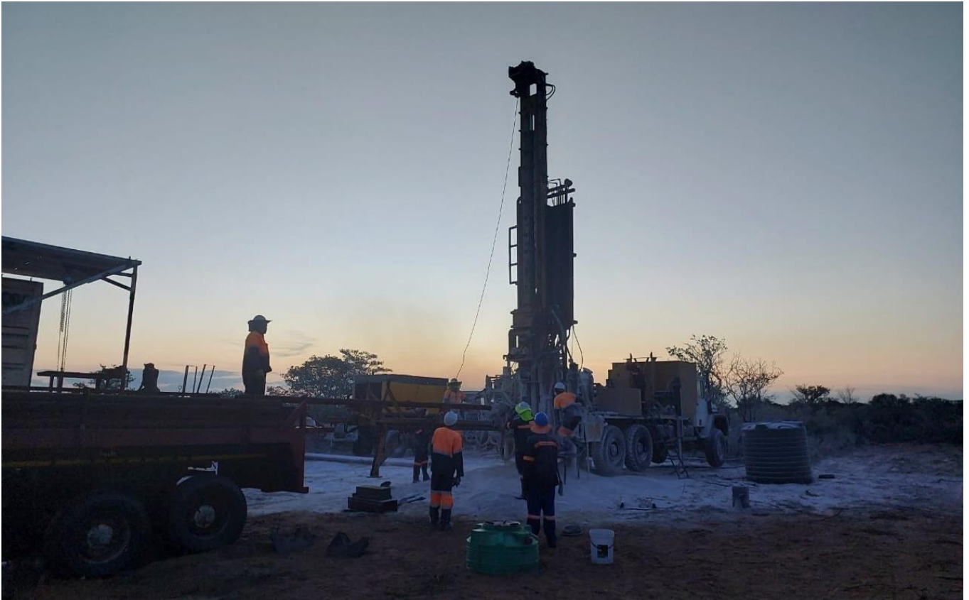
Figure 3. Pitse Pilot well 3.5B being spudded. (Source: Botala)
