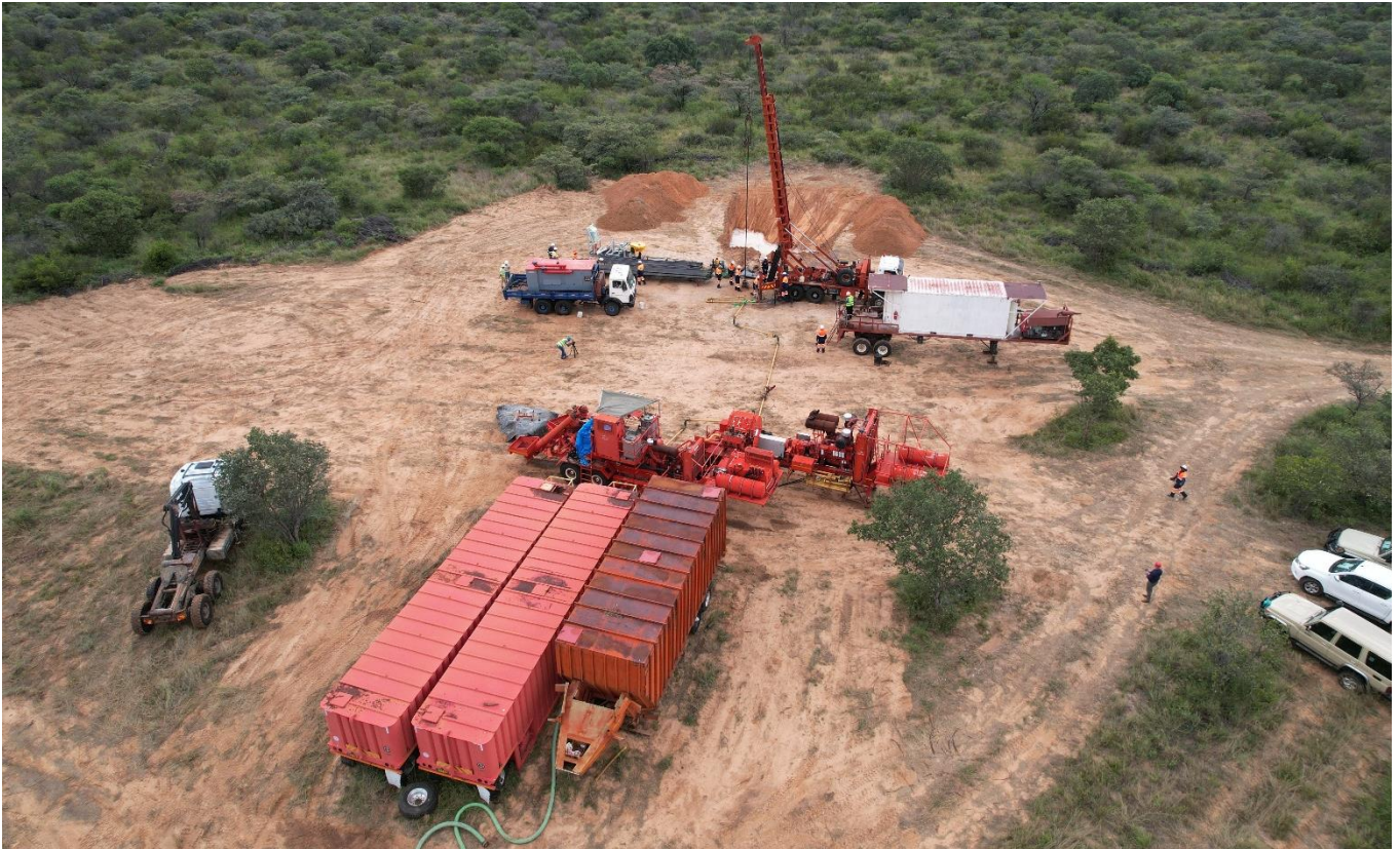
Figure 1. Pitse Pilot well S3.3 perforation and jetting operations. (Source: Botala)
